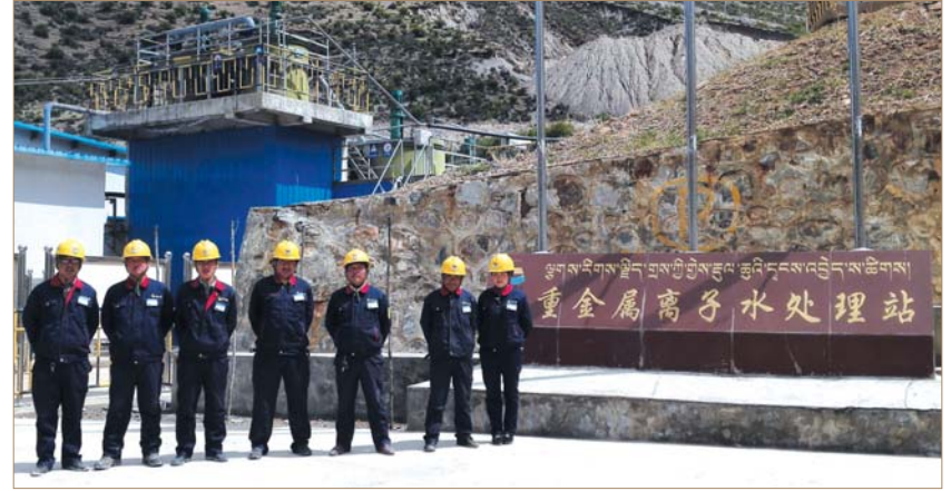
Tibet Huatailong's treatment facility for heavy metal cation containing water
