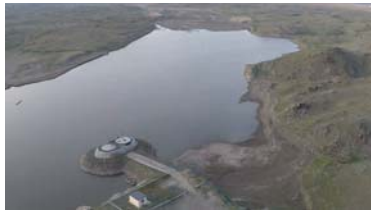
Reservoir in Inner Mongolia Pacific Mining Co Ltd.
