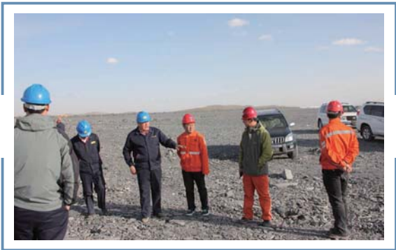
Zhang Lisheng, Chairman of Inner Mongolia Pacific, was carrying out a special inspection to the construction team
