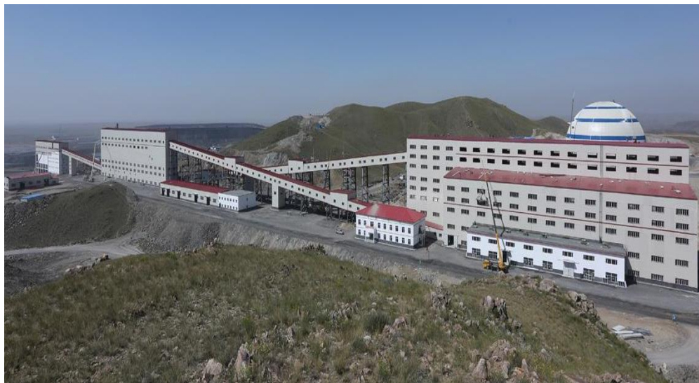
Panorama of the newly completed 30,000 tpd crushing system
