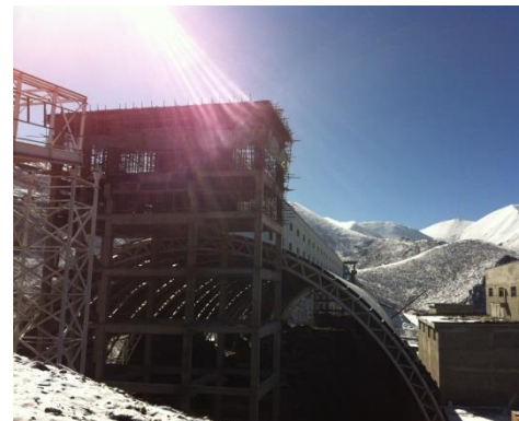
❖ construction of ore storage nearly completed
