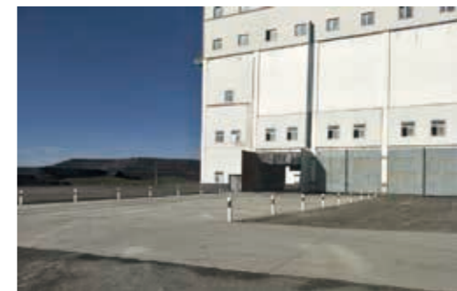
CSH reduced dust of the crusher workshop
