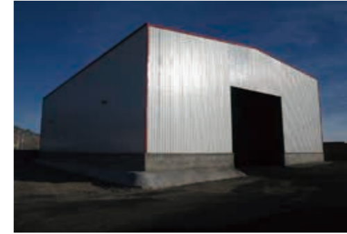
CSH built up new coal sheds to reduce dust
