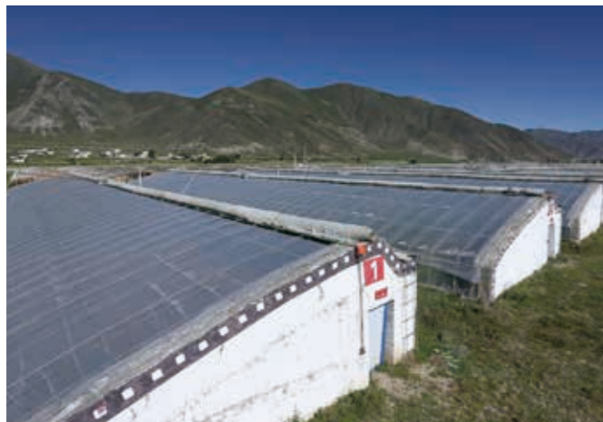
Vegetable greenhouse and vegetable base funded by Jiama Mine
