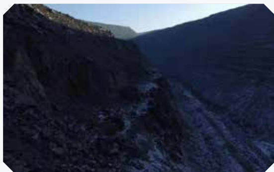
CSH Mine's drones monitored slope.
