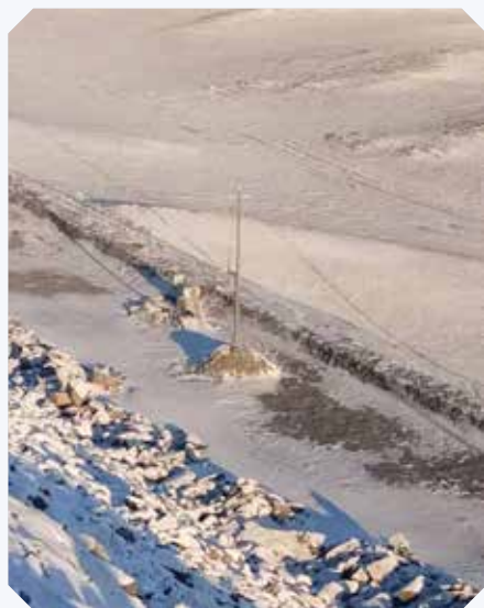
Water-holding dam built by CSH Mine
