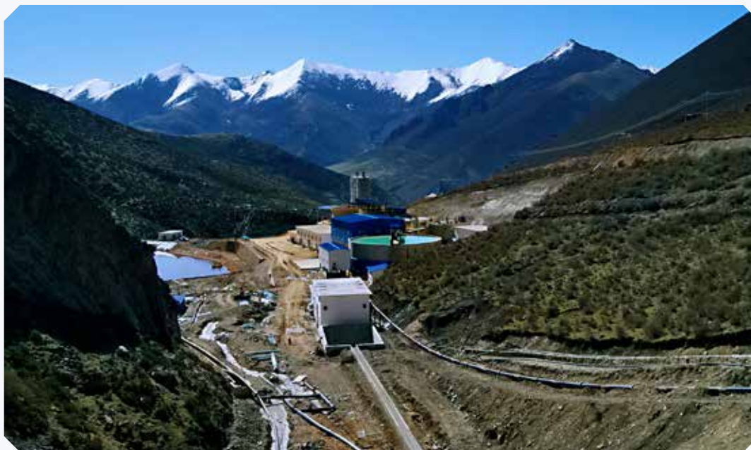
Jiama Mine invested in building Sibugou water treatment plant.
