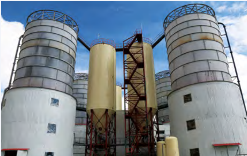
Backfill station at Jiama Mine
