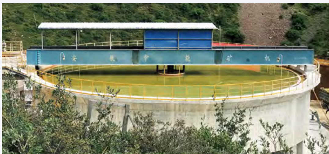
Jiama Mine invested 72 million yuan in constructing the sedimentation tank for iron removal of Sibü acidic spring water treatment plant
