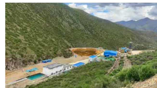
Jiama Mine built Sibugou water treatment plant.
