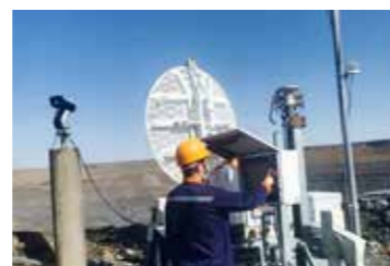
Radar monitoring system for slope stability in open pit of CSH Mine
