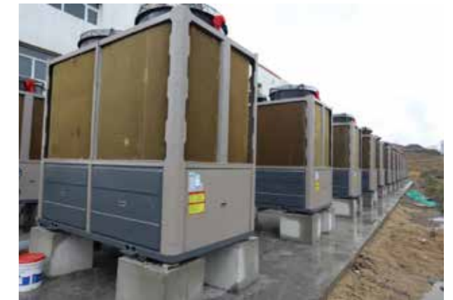
The air-source heat pumps system of CSH Mine
