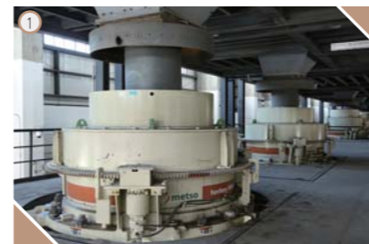
① HP800 gyratory cone crusher
