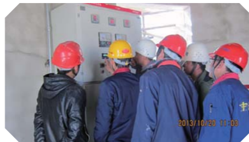
Tibet Huatailong organizing regular electrical equipment inspection
