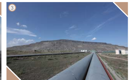
③ Heap leaching pad
