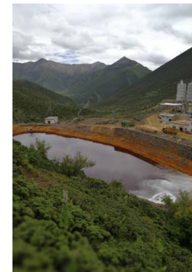
Jiama Mine built Sibugou water treatment plant.
